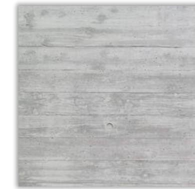
Horizontal board frame concrete (External walls)
